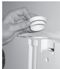
2. When using the original 42 mm polypropylene pipe, first place a washer to the hole. The installation can also be started with the corner pieces.
