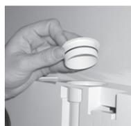
2. When using the original 42 mm polypropylene pipe, first place a washer to the hole. The installation can also be started with the corner pieces.
