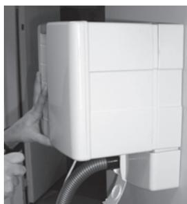
5. Place the central unit directly towards the filter unit. Make sure that the rubber pieces behind touch their counterparts.
